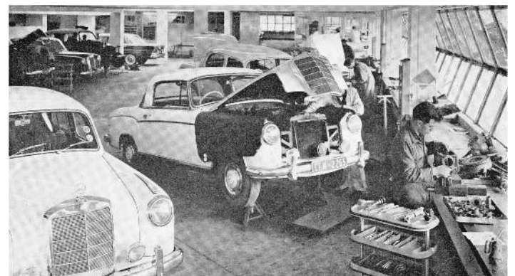
A section of the workshops, note the cantilevered windows above the work bays
